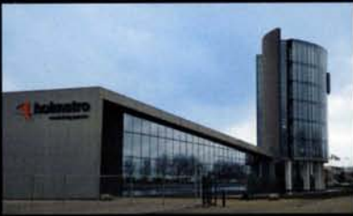
Holmatro N.V. World Headquarters Raamsdonksveer, The Netherlands
